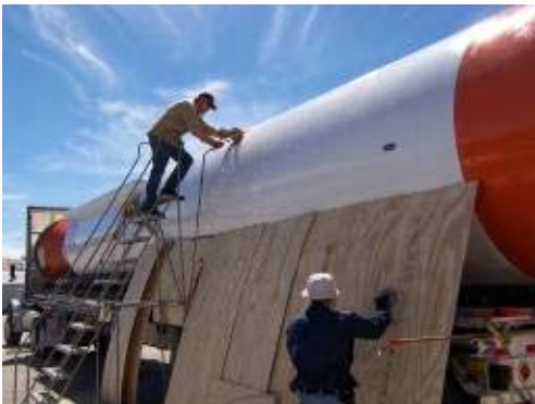
Preparing for Drop: Cutting Away Hoist Attachment Points
