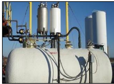
Propane Conditioning Tank
